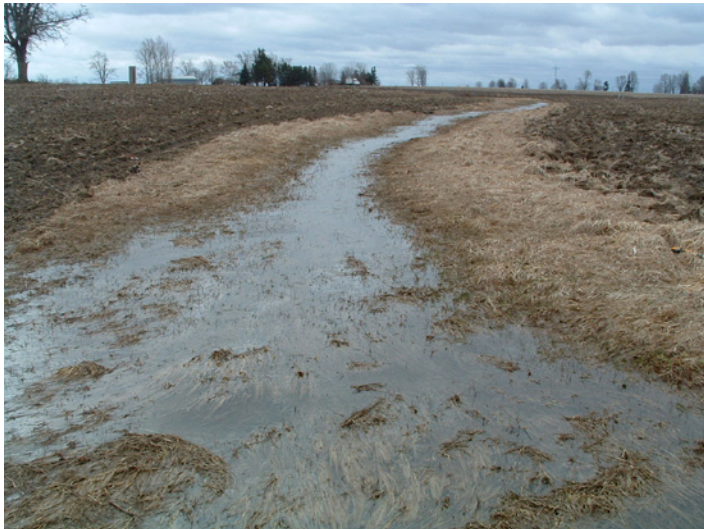
This grassed waterway was installed through the CWP to protect the farm field from soil loss during spring snowmelt and rainstorm events.
