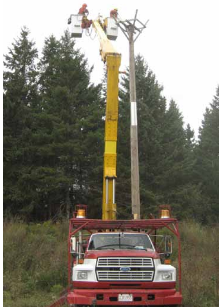
The London Hydro crew erect the new nesting platform and tower.
