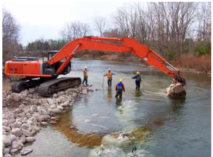
Protective stone is placed around the exposed watermain.
