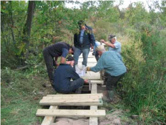
The boardwalk project nears completion.
