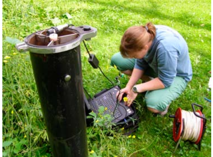
Downloading data from a groundwater monitoring well.
