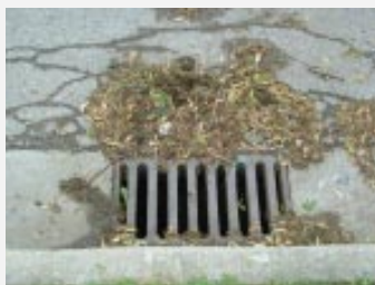
Catchbasins with lots of vegetative material are prime breeding sites for WNV mosquitoes.
