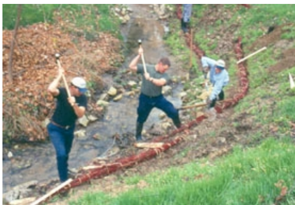
Bioengineering work on a steep river bank in Lambeth
